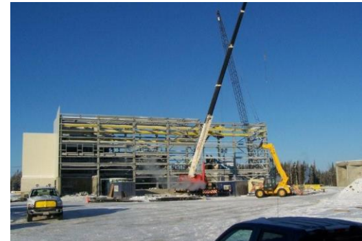
Construction of Mill Building (2008)
