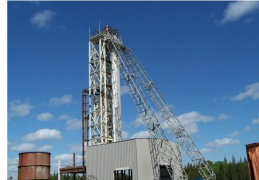
Construction of Headframe (2008)
