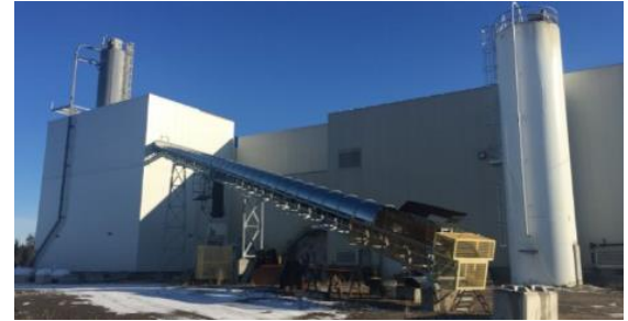
Paste Backfill Plant completed in 2012
