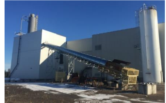
Paste Backfill Plant (2012)
